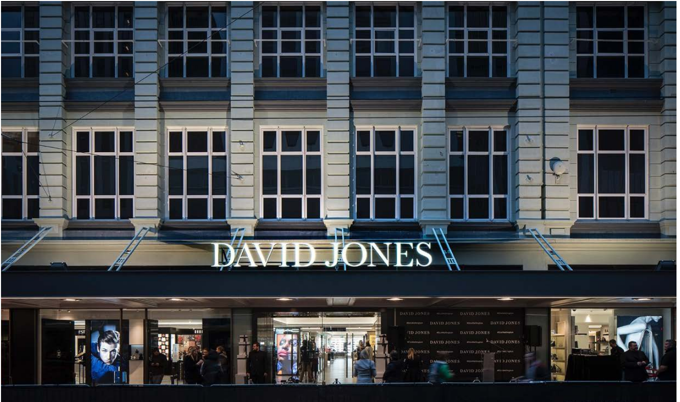
David Jones, Wellington now stands within a heritage building in Wellington's CBD
